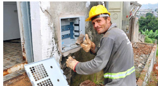
New water connection is completed in Itaquaquecetuba
