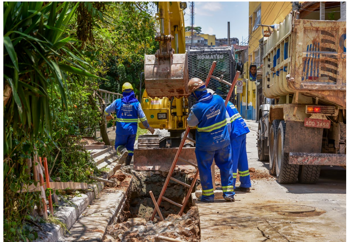
New Pinheiros River Program workers install collecting networks in the Alto Pirajuçara basin, in São Paulo
